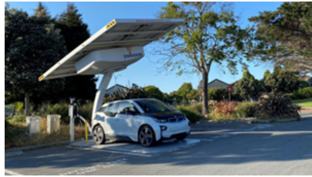
A 2020 photo from Marina Bay Park in Richmond showing a solar-powered electric-vehicle charging station.
